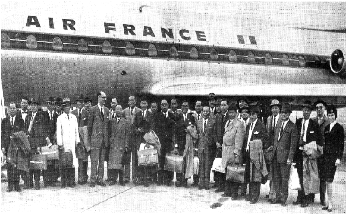
ON OFFICIAL TOUR: Top ranking officials of the National Defense College of Thailand made an official tour of Europe recently, visiting Italy, Germany, France, England, and the Scandinavian countries. The group is shown ready to board an Air France Caravelle jetliner at Orly International Airport for the flight from Paris to London.
